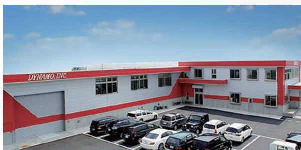
■ Main Office Dynamo, Inc.
